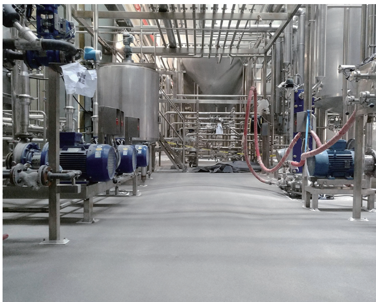
Sand-Broadcast Anti Slip Waterborne Polyurethane Mortar system 3mm
